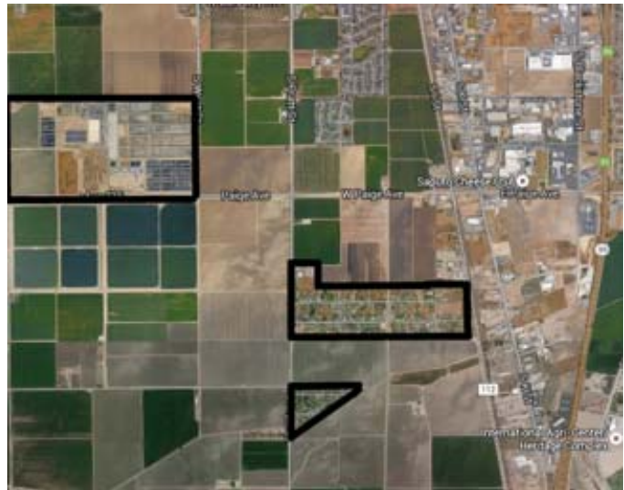
View of Tulare’s wastewater treatment plant (outlined in upper left corner) and Matheny Tract (outlined in lower right). The diagonal route right of Matheny Tract is the railroad referred to by Dorman. (Google Earth)
